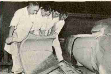
After plaster has set, cast is removed.
