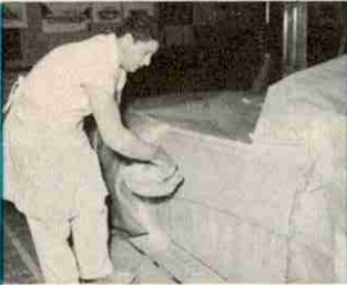
Thin plaster solution is slung on first, followed by thicker mixtures.
