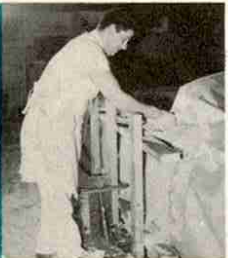
Wood frame is attached to cast by strands of soaked hemp.
