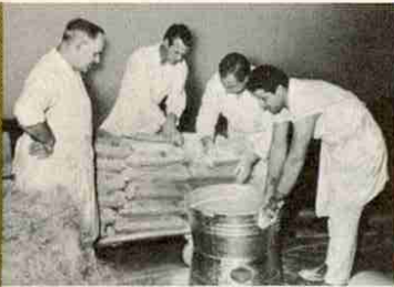
Plaster, water and Manila hemp are readied.
